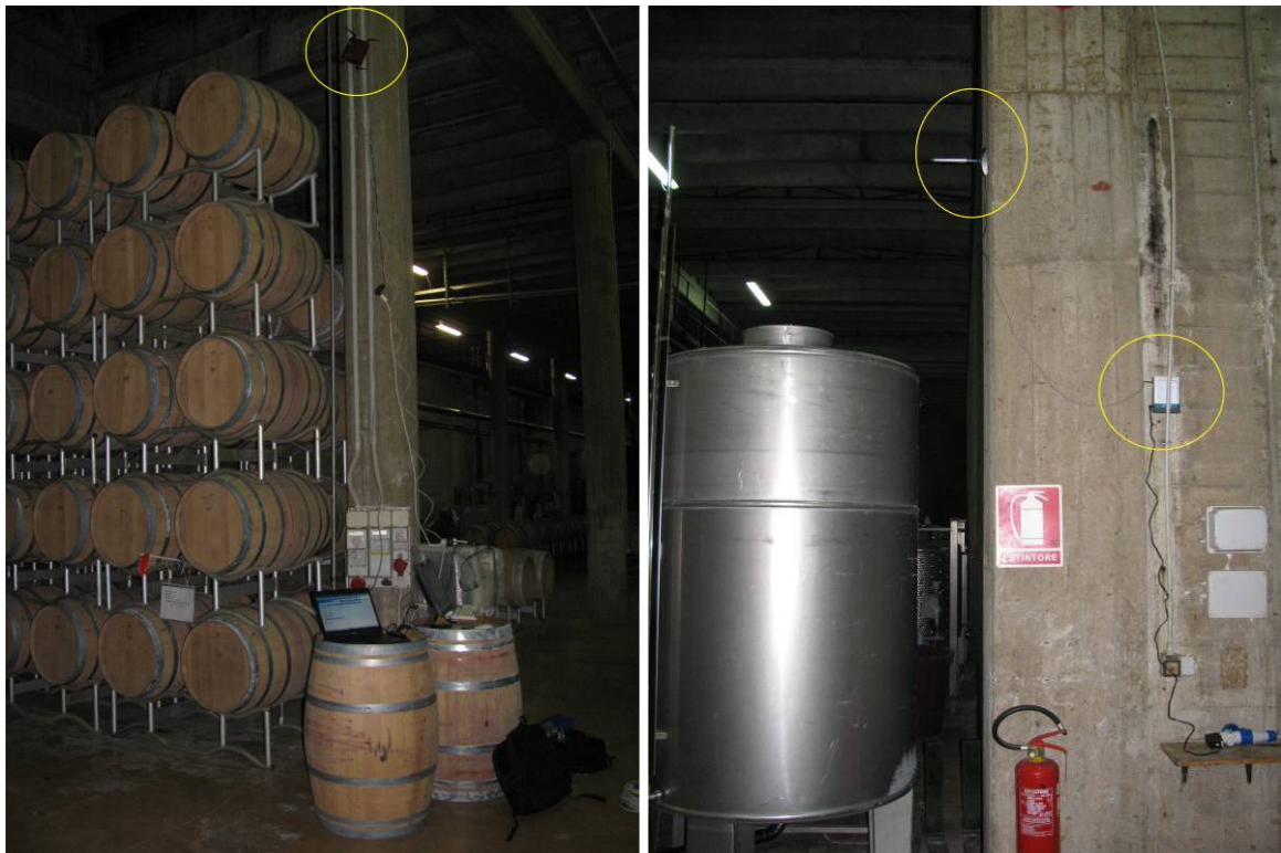
Figura 33: access point in barricaia
